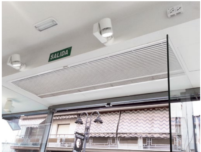
Recessed Dam Model with exposed inlet grille
